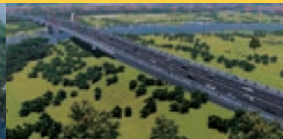
Kabayani St.-Matandang Balara Bridge
