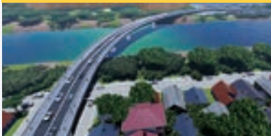
Marcos Highway-St. Mary Ave. Bridge
