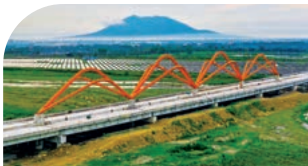
The 900-meter Sacobia Bridge is part of the ANAR. The entire ANAR was opened in February 2024.
