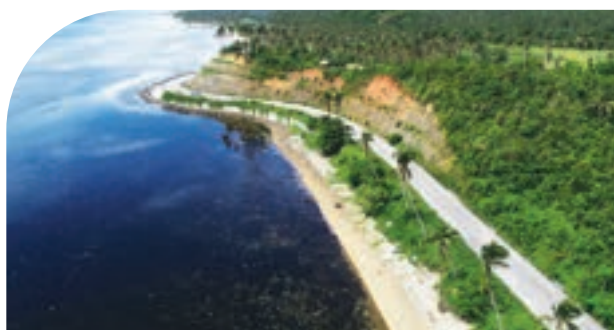
The Matnog-Sta. Magdalena-Bulusan Road provides easy access to declared tourism sites in the municipalities of Matnog, Sta. Magdalena, and Bulusan in Sorsogon. This PhP1.36-billion road was completed in April 2023.
