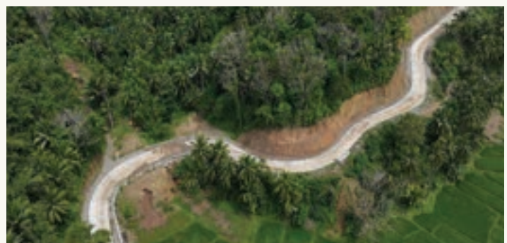
A two-lane FMR stretches from Brgy. Lumbang Este to Brgy. Marigondon in Cajidiocan, Romblon. It was completed in October 2023.
