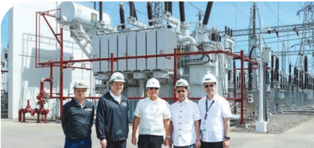
The President, with DOE Secretary Raphael P.M. Lotilla and officials of the National Grid Corporation of the Philippines (NGCP), inspects the Bacolod Substation prior to the Ceremonial Energization of the Cebu-Negros-Panay (CNP) 230-kilovolt (kV) Backbone Project on April 08, 2024.
